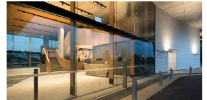
AVEO, BELLA VISTA - STRONGBUILD
