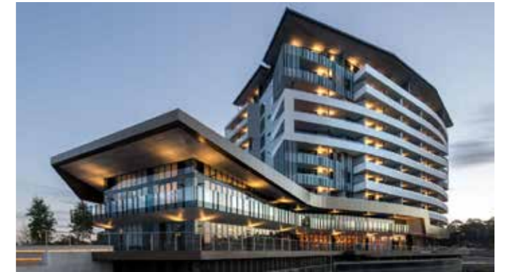
AVEO, BELLA VISTA - STRONGBUILD
