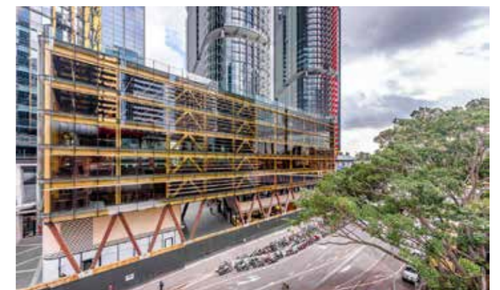
INTERNATIONAL HOUSE, SYDNEY (TZANNES ARCHITECTS)
